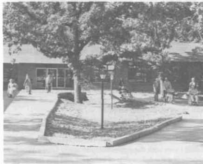
New conference and retreat center in Walworth, Wisconsin.
