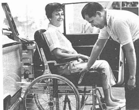
"Seymour engages the slides to the bucket seat mounted on the carriage."
