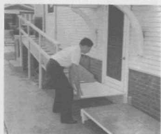
HINGED "DRAWBRIDGE" across side entrance is swung back onto ramp when latter is not being used so that door can be opened without interference
