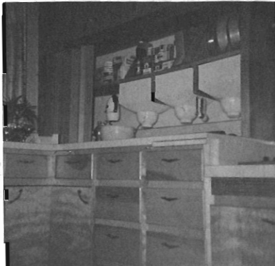
(r) Oven doors are French - no reaching over a hot oven door. Cooking utensils are hanging in big drawers under burners. There is also a part which drops down over the burners.
