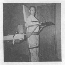
board of bed. With it in place, and bed ten degrees low at foot, two people can easily slide me onto it. I am strapped fast, and foot end allowed to ride on floor, as foot of bed is turned up by turning belt by hand. Two people can swing board up on a stool, remove straps, then on up and am slid down hill, back on to bed. Standing board is then removed, footboard folded, and stored under bed. Folding armrests support arms while standing.
